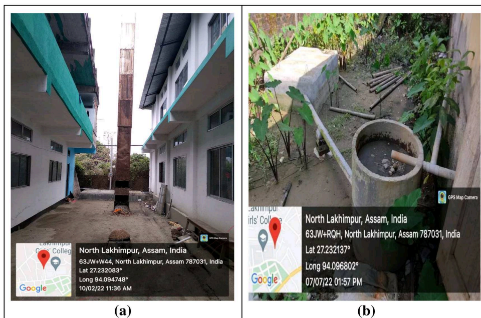
Figure 8: (a) Incinerator (b) Liquid waste management facility
